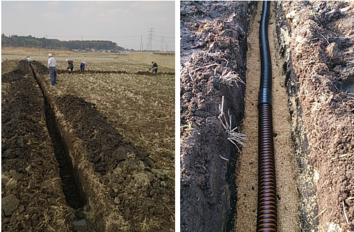
Fig. 3.10 Picture of embedding culvert in volcanic ash soil paddy field (Date taken 17-March 2014)
