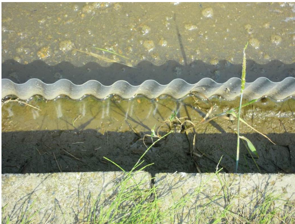
Fig. 3.7 Picture of levee covered by polycarbonate borders (Date taken 4-June 2013)
