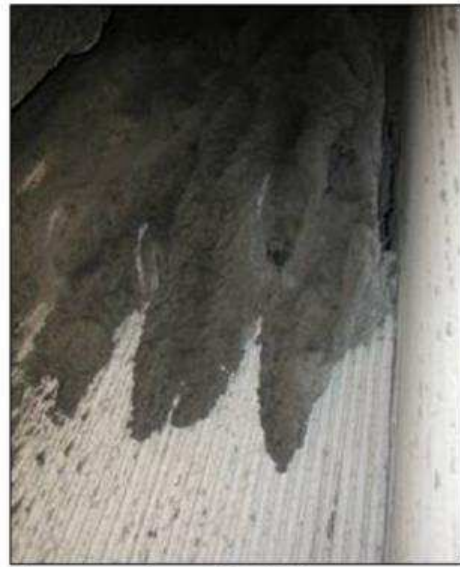
Screen tubes AFTER approx. 14 days of operation
