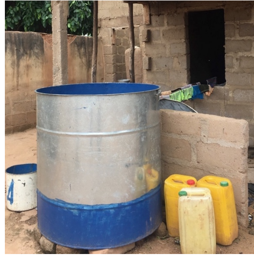
Photo 6 Shared water tank in compound
