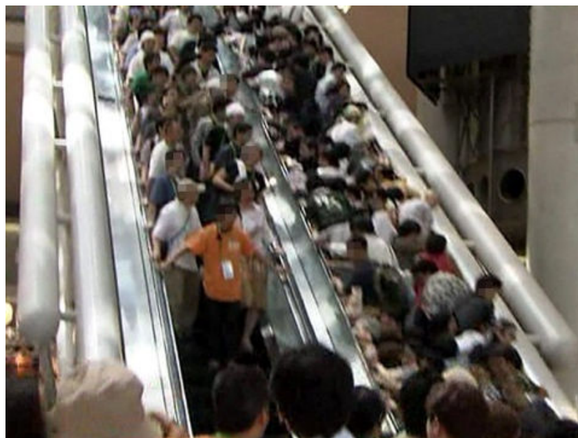
Fig. 1.7 Escalator reverse run accident by loose bolt 21)
