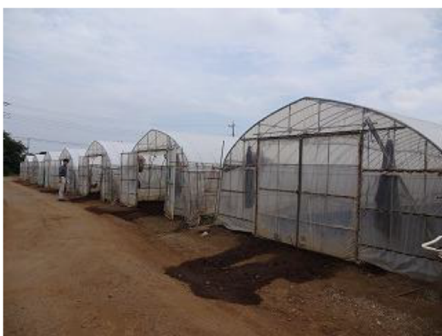
Fig. III-1. Green houses where this study was conducted.
