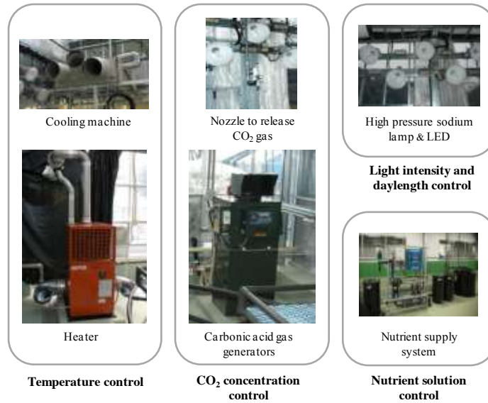
Fig. 1.7. Controlling equipments that are used in the blueberry factory, Tokyo University of Agriculture and Technology (Source: Ogiwara and Arie, 2010).
