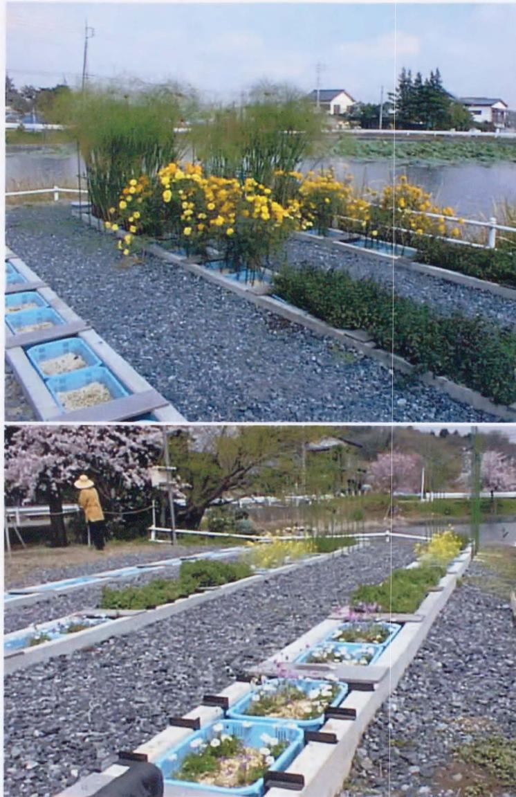
Plate 7-2. Plant bed filter ditch near Konda Pond.
